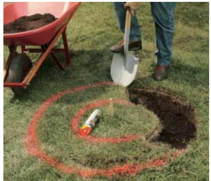
A. Outline the location of the footing using spray paint and a piece of string. Then dig a circular trench 10" deep.
