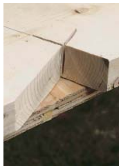
C. Cut the bird's mouth by overcutting the lines just until the blade cuts entirely through the board.
