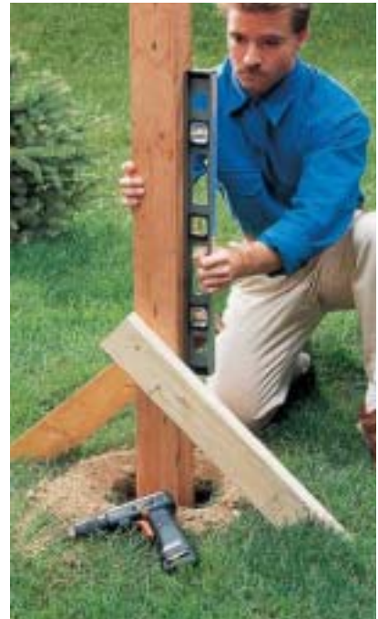
C. Position each post in its hole. Brace the post with scrap pieces of 2 x 4 on adjacent sides, and adjust it until it is plumb.
