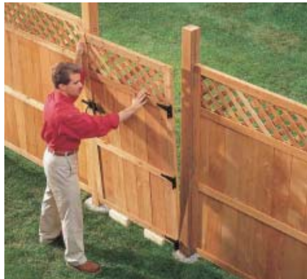
D. Attach three evenly spaced hinges to the gate frame. Shim the gate in place and attach the hinges on the gate post. Attach the latch hardware to the gate and then to the opposite post.
