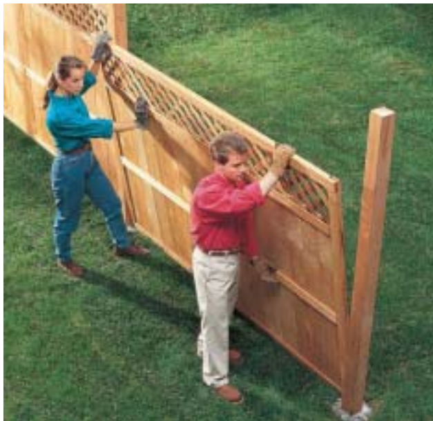
A. Lay out the fence line and set the posts. Test-fit a panel and outline its position on the inside faces of the posts.
